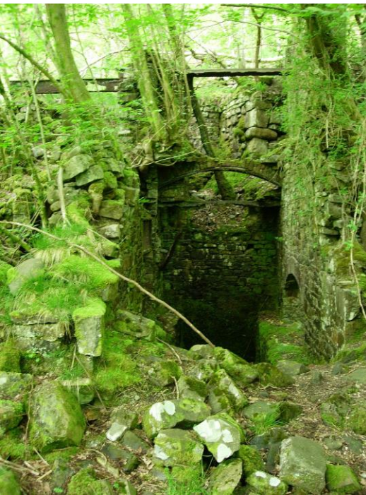
Old crushing plant for one of the silica mines, wheel pit.
